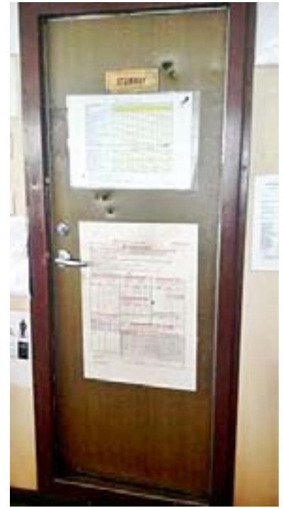
Damage to the bridge of SP BRUSSELS from the firefight on the bridge. (Source: withheld)
